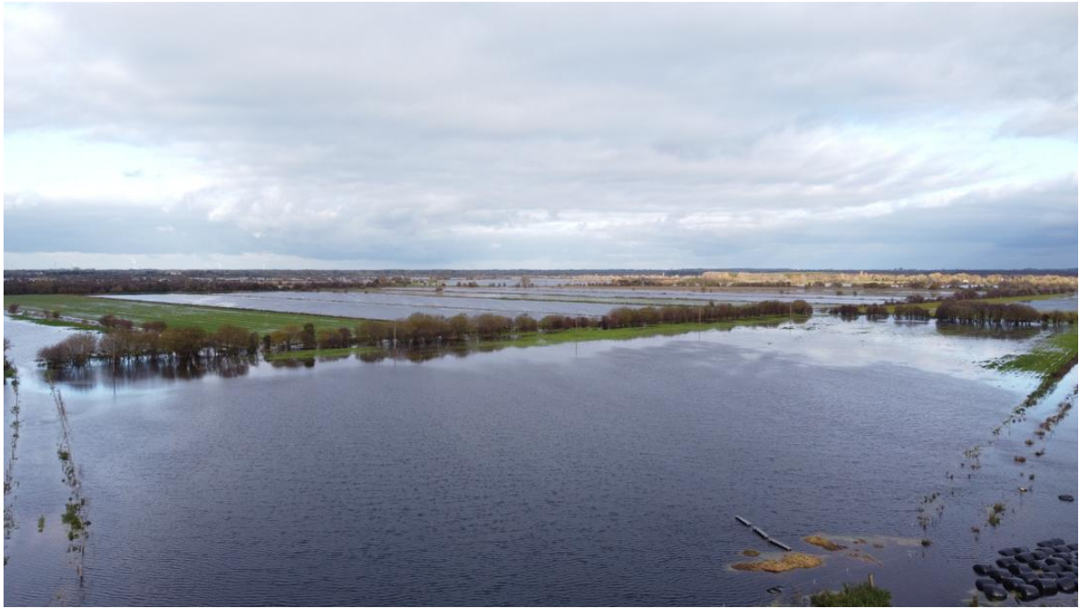
Photo29: Taken on the 16/11/25 after the heavy rainfall.
