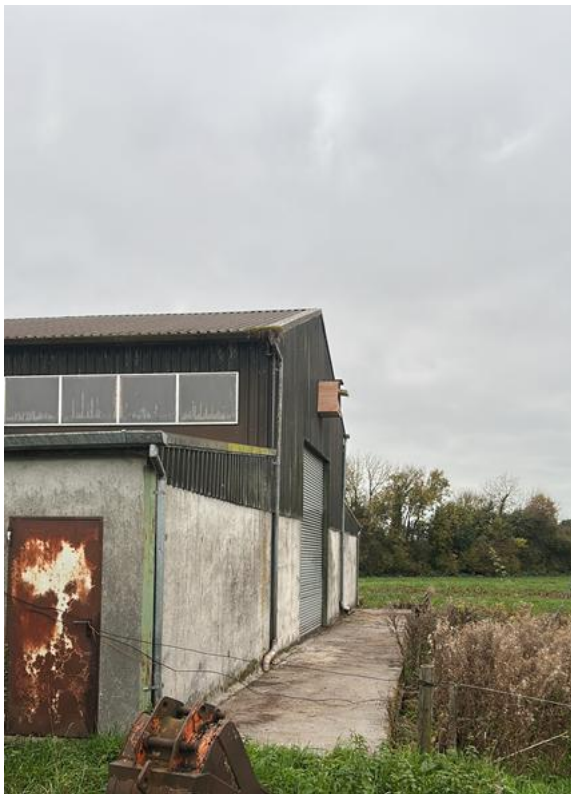
Photo54: One of our Owl Boxes located on the structure that is 355 m from proposed Turbine 1 (ITMx 660271, ITMy 714701)
